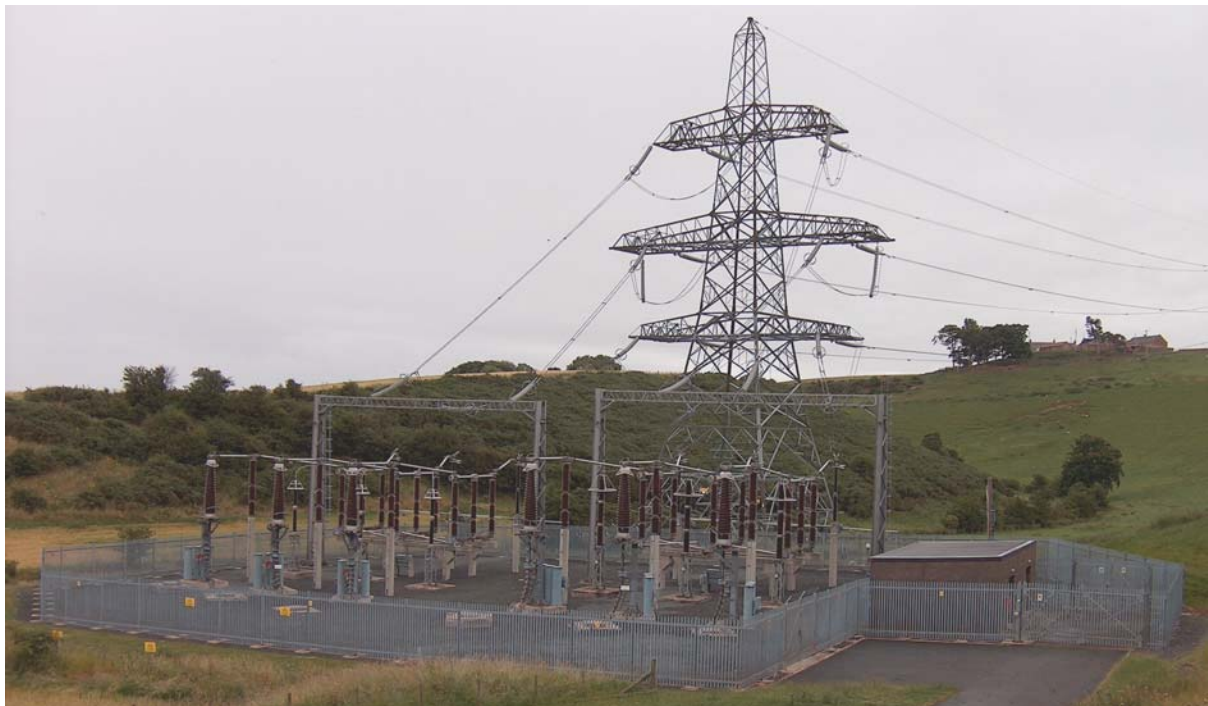
▲ Sealing end compound (smaller than the proposal would require) and terminal tower at under-grounding terminal.
